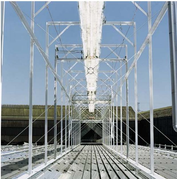
Fig. 10: Flat mirrors concentrate sunrays on receiver tube
