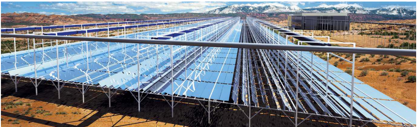
Fig 9: Suggested decentralised power generation for a farm in southern Egypt. 80 000 m² reflector area to produce electricity, desalted water and cooling supported by shadow for farm inhabitants, animals and food processing industry (Source of graph: FHG-ISE)
