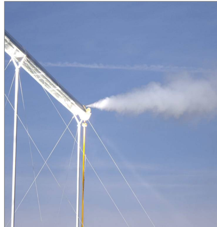
Receiver showing steam generation at demonstration plant in Spain
