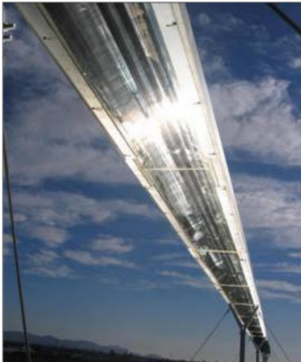
Receiver showing steam generation at demonstration plant in Spain
